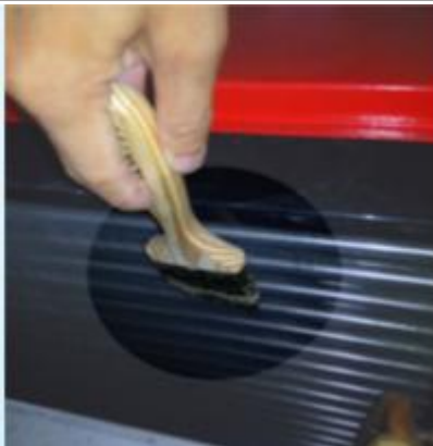
3. The banister brush is used along the vertical fin (up or down). It is noted that the fins are very sharp, so the gloves must be worn during the operation.
